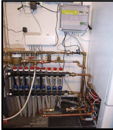
Figure 9.2: One of the 54 domestic heat pumps subsequently installed with sensors and actuator that can be accessed over an Internet connection.
