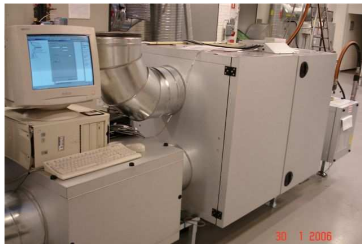
Figure C.1: HVAC test system
