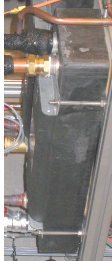
Figure A.5: The evaporator.
