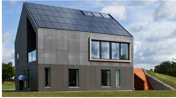
Figure 11.3: Energy Flex House: a low energy building for testing, developing and demonstrating innovative energy efficient solutions
