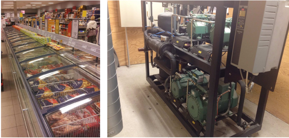
Figure 6.7: Fakta supermarket used for the “PowerCap” experiment (The cold storages and the compressor rack)
