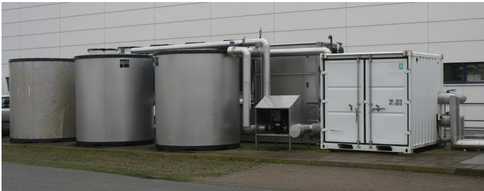
Figure 6.8: Grundfos chiller with the ice storages
