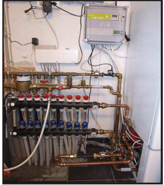
Fig. 2. One of the 54 domestic heat pumps subsequently installed with sensors and actuator that can be accessed over an Internet connection.
