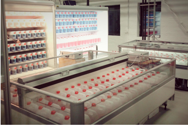
Fig. 2. The medium temperature section of the supermarket refrigeration system with foodstuff replicas.
