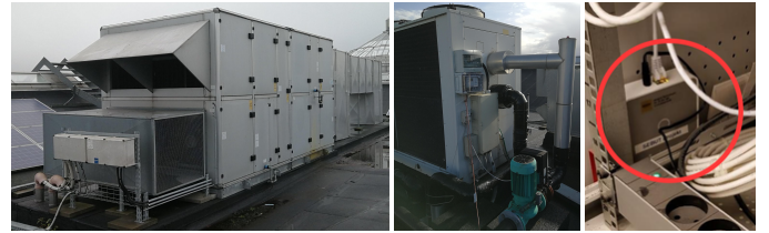
Fig. 1. From left; AHU, chiller unit and Building Management System (BMS) gateway for remote data acquisition and control, situated at Kolding Storcenter, a Danish shopping center.
